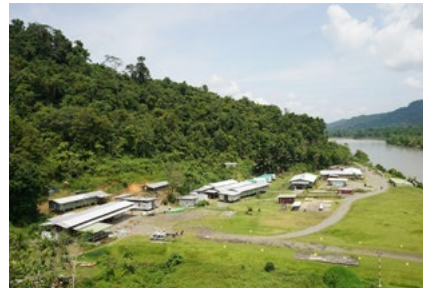
AN AERIAL VIEW OF THE FRIEDA RIVER COPPER-GOLD PROJECT SITE FACILITIES AT THE FRIEDA RIVER AIRSTRIP.
